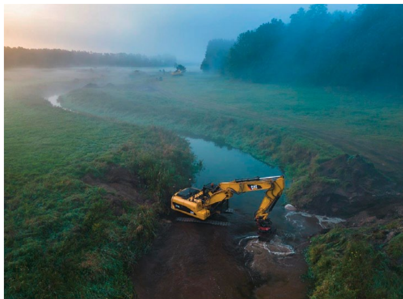
Construction of gravel prisms in the Ina river Anlage von Kiesdepots in der Ihna © Neil Aldridge/Rewilding Europe
