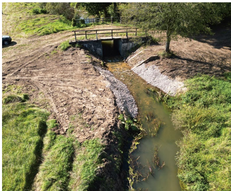
New gravel depot in the Perznica Neutralized migration obstacle at Perznica river Neues Kiesdepot in der Perznica Neutralisiertes Wanderungshindernis am Fluss Perznica © Thomas Winter © Thomas Winter
